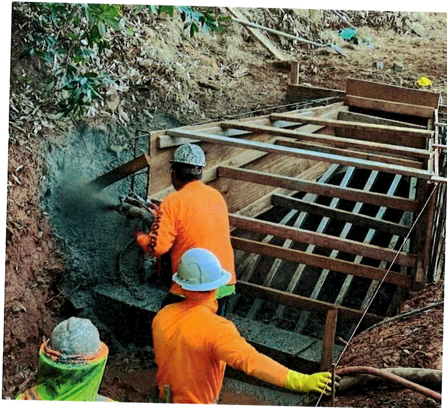
Headwall During contruction
